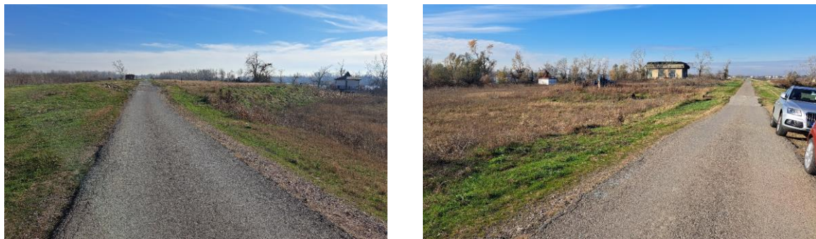
Figure 2-5: Existing access road on the embankment
