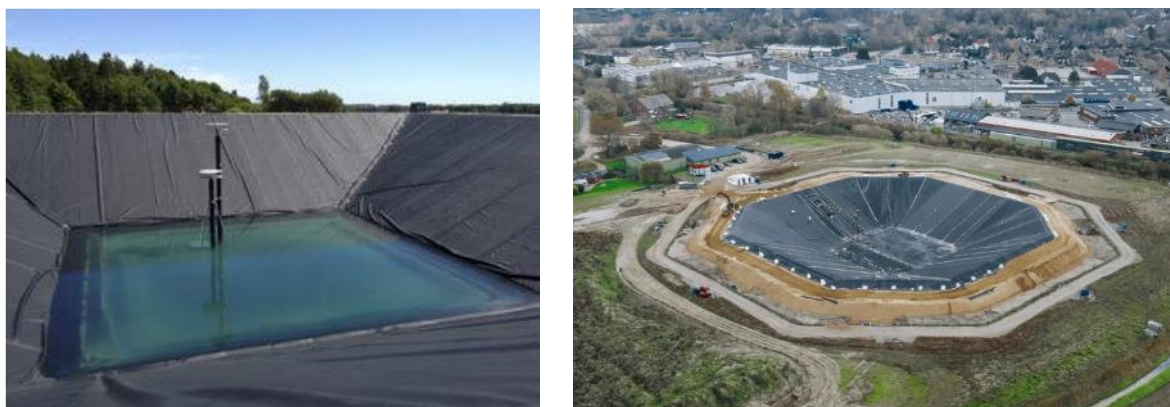
Figure 2-6: Examples of PTES layout
